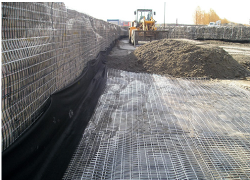
Figure 9. Anchored gabions
