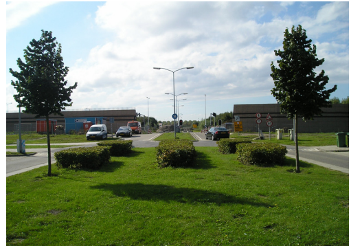
Figure 10. View of the two earth structures
