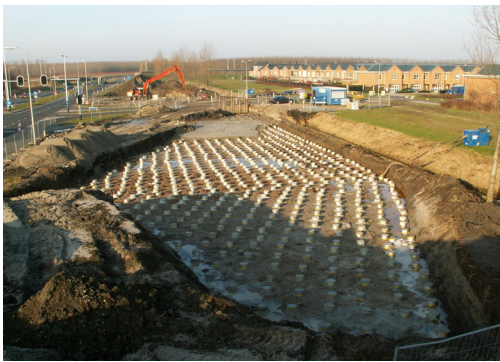
Figure 8. Pile foundation
