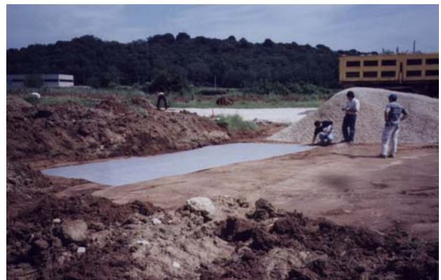
Figure 1. On site work phases
