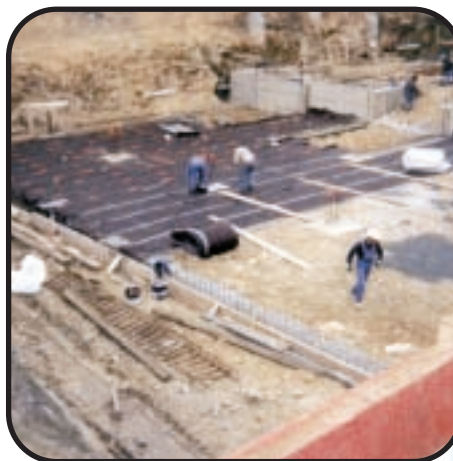
Vannes, France Parking enterré
