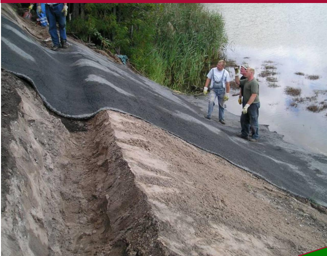
Above: Eroded slope before installation of Enkamat A20
