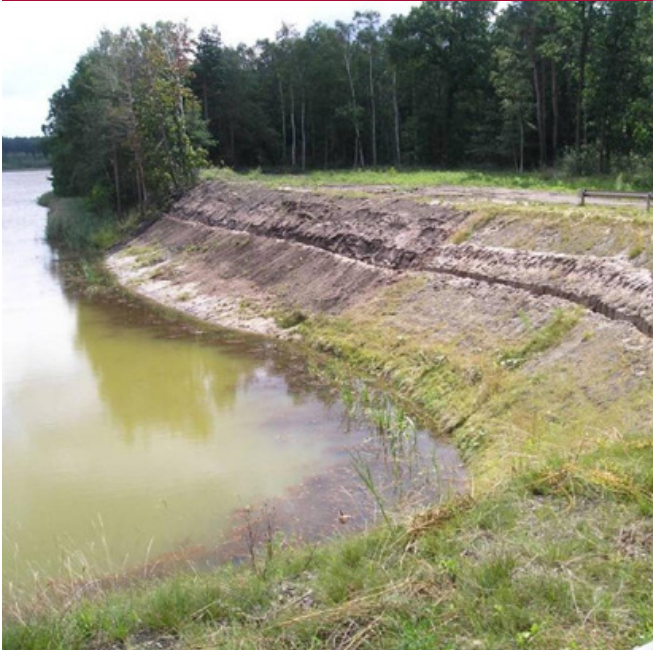
Above: Eroded slope before installation of Enkamat A20
