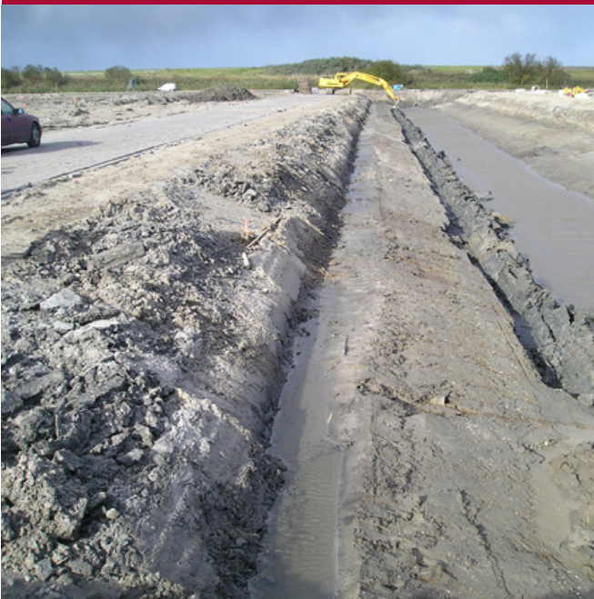
Above: Creating the channels at the top and bottom of the slope Below: Fitting of Enkamat A20
