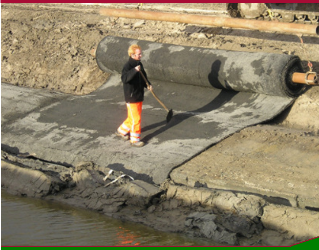
Above: Creating the channels at the top and bottom of the slope Below: Fitting of Enkamat A20
